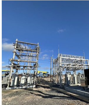
New Bus (Right) and Bus for demolition (Left) at the Old Perlican Substation.
